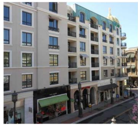
Designed by Togawa Smith Martin, Inc., The Americana in Glendale, Calif., includes five stories of wood-frame construction over a concrete podium and two levels of subterranean parking. Photo by Michelle Kam-Biron
